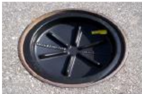
Figure 18 - Inflow Defender Manhole Rain Dish.
