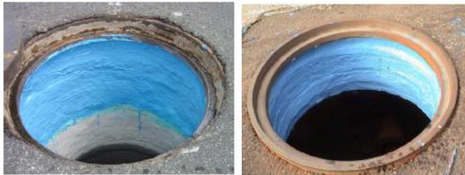
Figure 16 - chimney seal installed.
